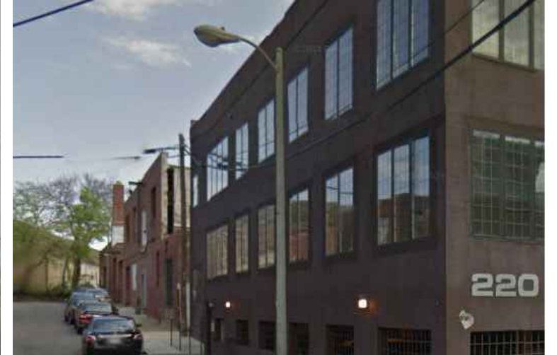
4 EXISTING COBRAHEAD STREETLIGHT
