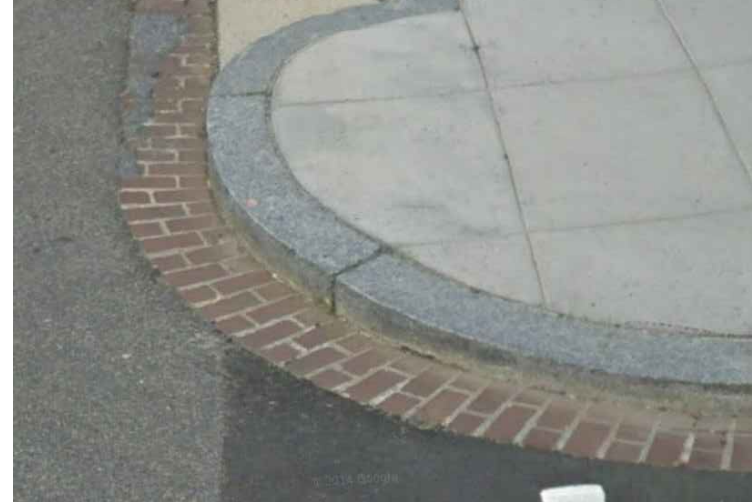
3 DDOT GRANITE CURB AND BRICK GUTTER
